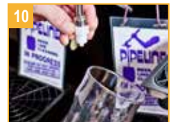
10 Remove dispense tap fittings, place in glass
