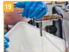
19 Flush out cleaning solution with a minimum of 10 litres of water per line
