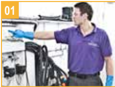
01 Turn off the cooler (Ideally 2hrs in advance)
